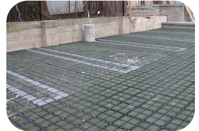
Install permeable pavers
