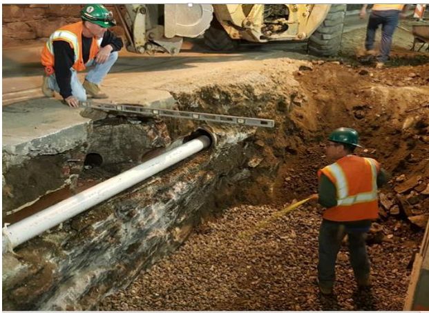
New below grade drainage system was installed in tunnel.
