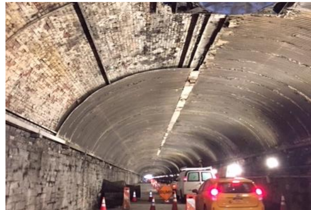
Corrugated metal ceiling panels are removed from the tunnel roof during asbestos abatement.
