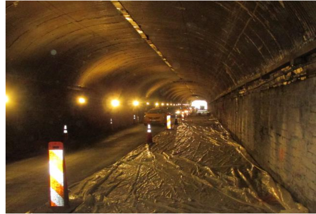
West side of the tunnel is prepared for installation of new roadway.
