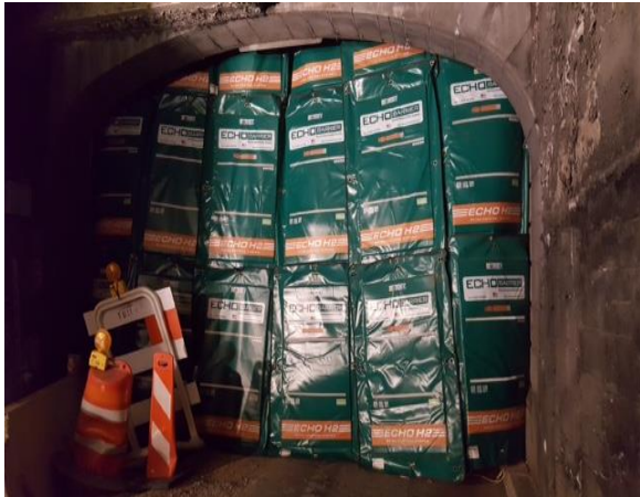
Noise reducing blankets cover the tunnel entrance at E. 33 rd Street.
